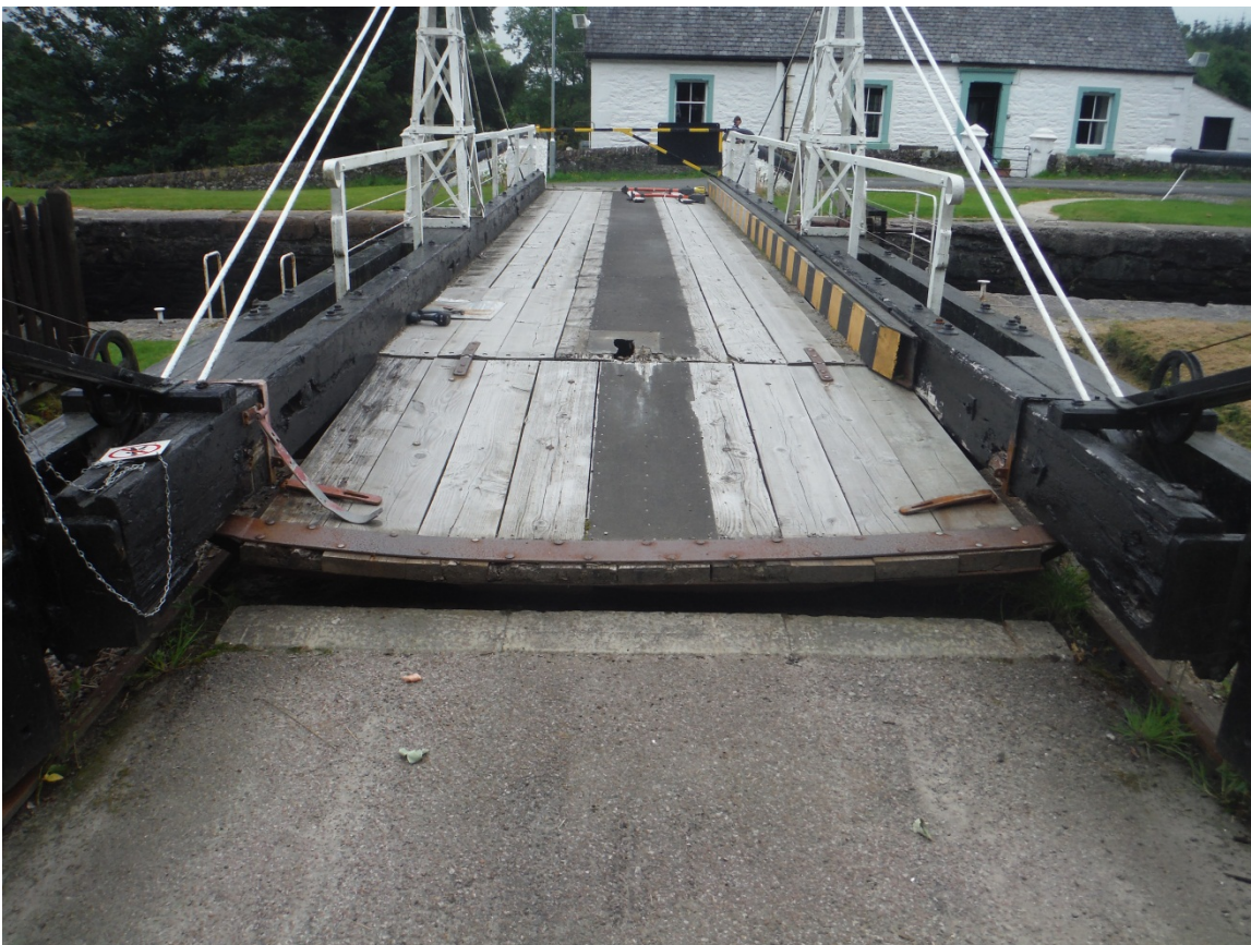
Deformed ramp section in raised position
