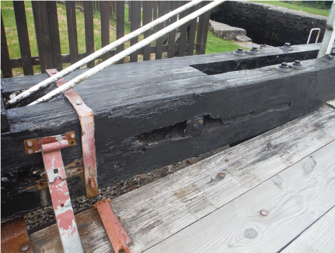
Decayed end of beam MB4
