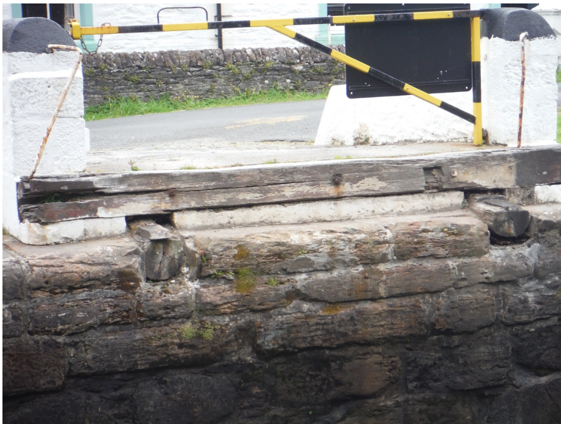
Uneven wear of timber supports and deteriorated timber 'log' supports at the north abutments
