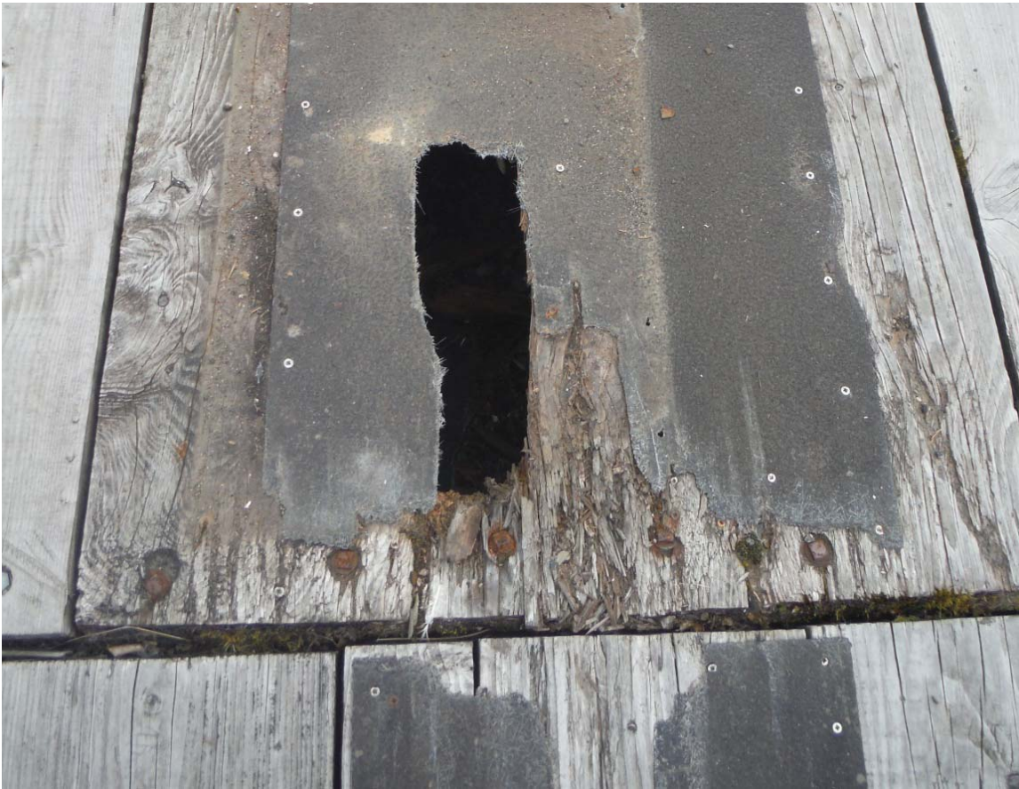
Decayed deck section underneath non slip central strip
