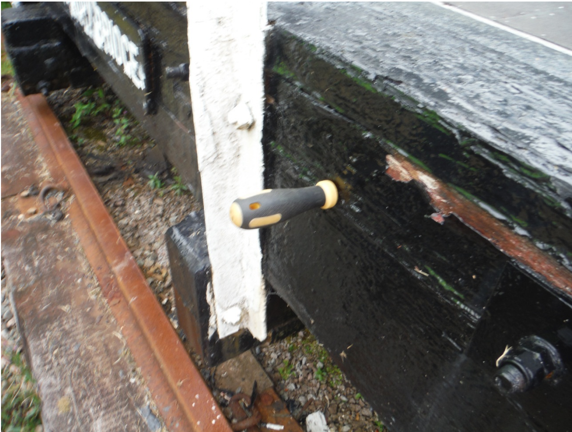
Decayed timber section in beam MB3
