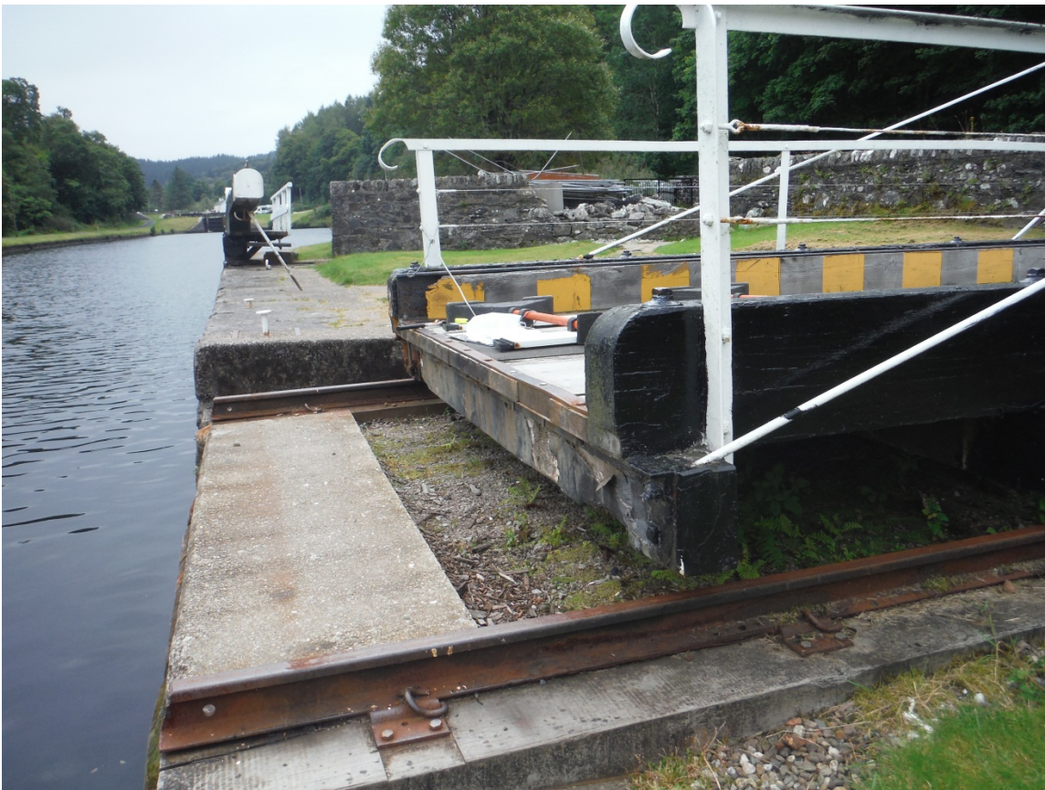
Front transverse beam showing distress. Timber sleeper split below the rail at the east end
