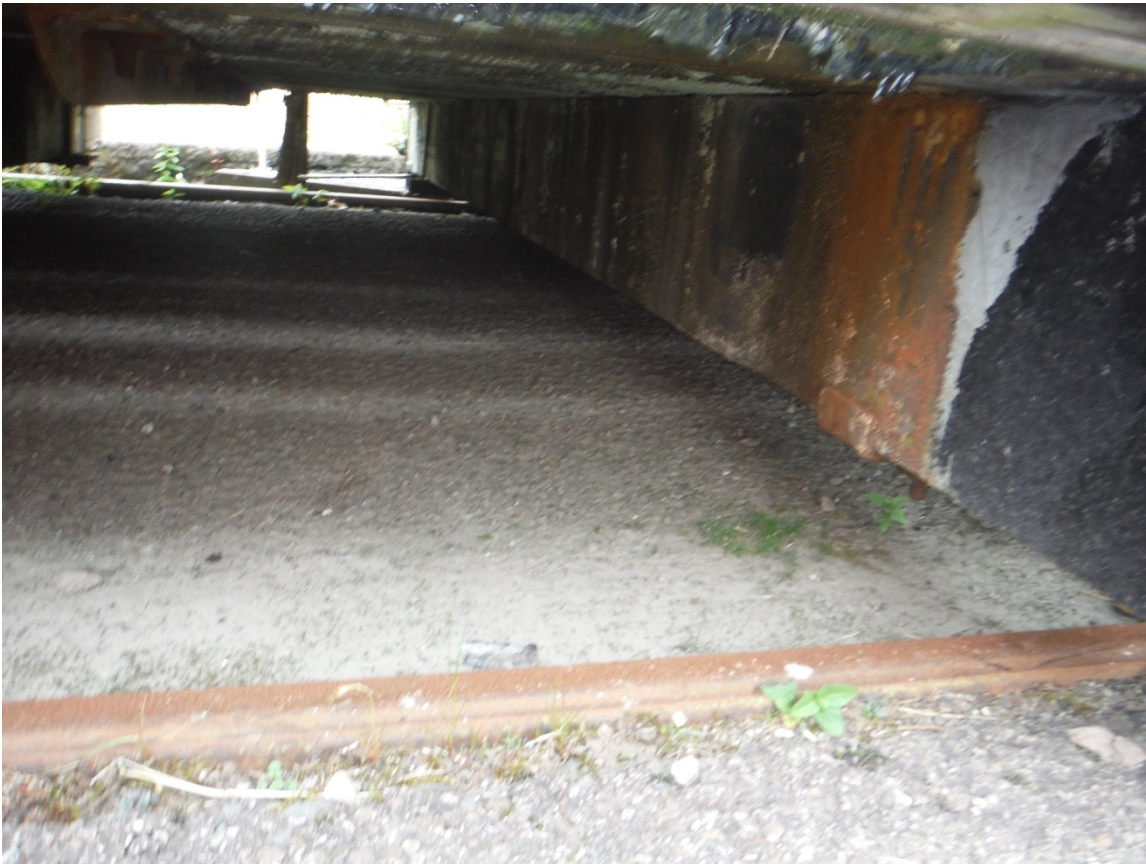
Transverse beam staining
