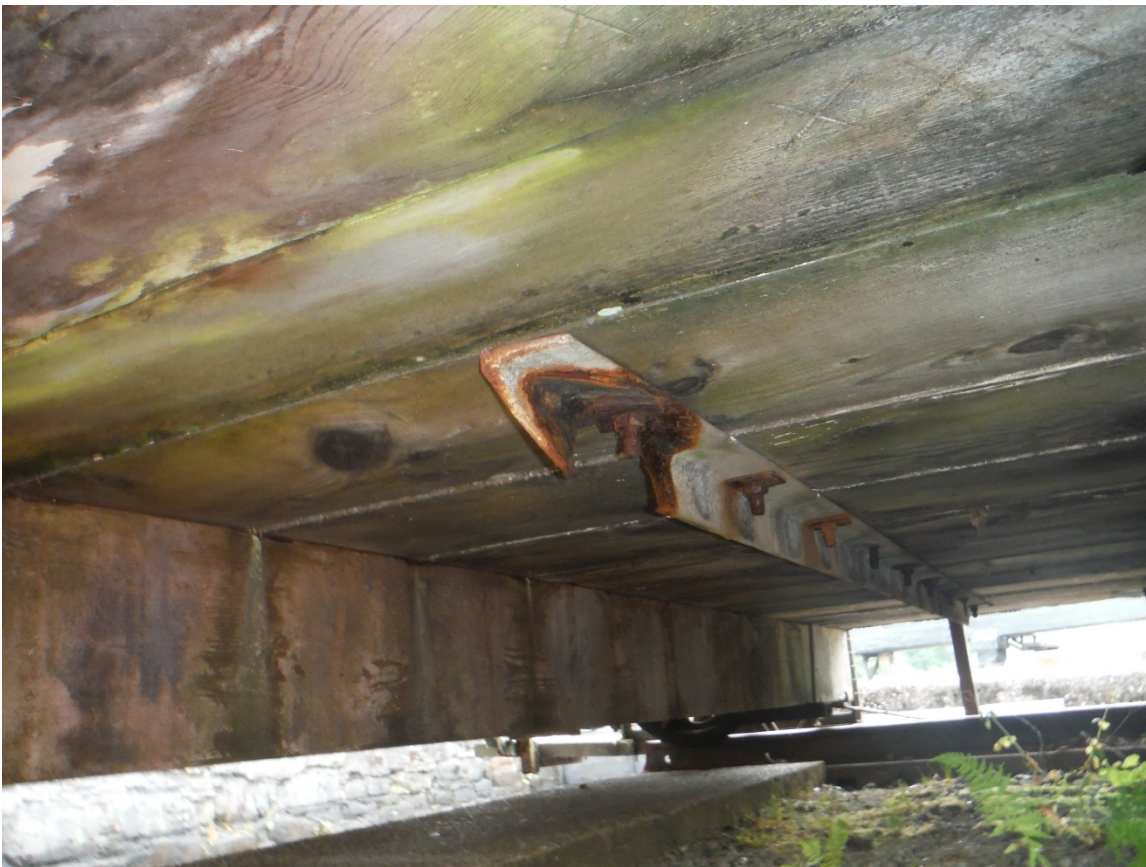
Loss of section at angle deck stiffener and corroded bolts
