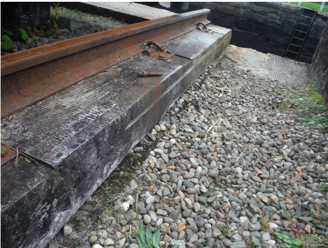
Friction marks caused by driving mechanism along the timber sleeper east face
